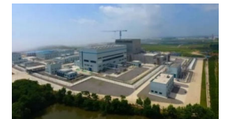
HTR-PM , China, 2x110 MWe HTGR in operation
