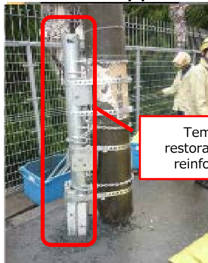
<Image of temporary restoration of utility poles>
